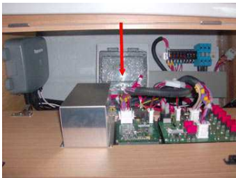
Decompounded switch 40A - Back of electrical panel
