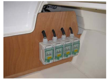
Bipolar circuit breaker 32A (Ref 2)
