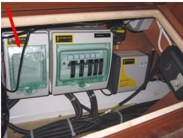
Differential switch 40A - Chart table unit
