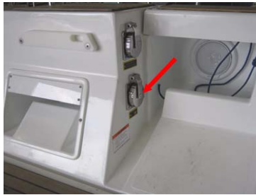
Shore power socket 220V - 32A (Ref 1)
