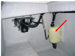
Hydraulic fluid tank
