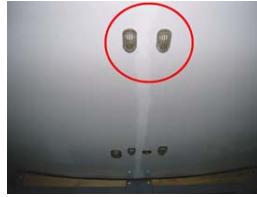
Layout of components Stuffing box - Seawater inlet
