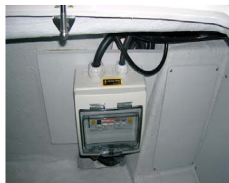
Differential circuit breaker (Ref 2)
