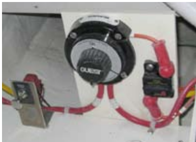
Generator Disconnect
