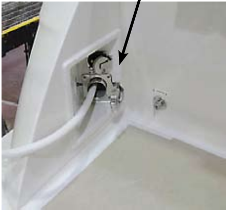
Shore Power - Aft Connections
