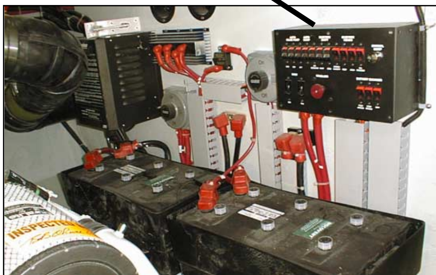
ENGINE ROOM AFT, STARBOARD BULKHEAD
