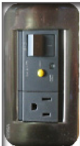
Ground Fault Circuit Interrupter (GFCI)
