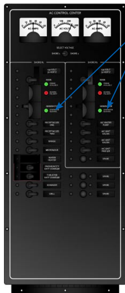
AC CONTROL PANEL
