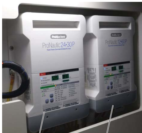
Accessory Battery Bank and Generator Battery Charger
