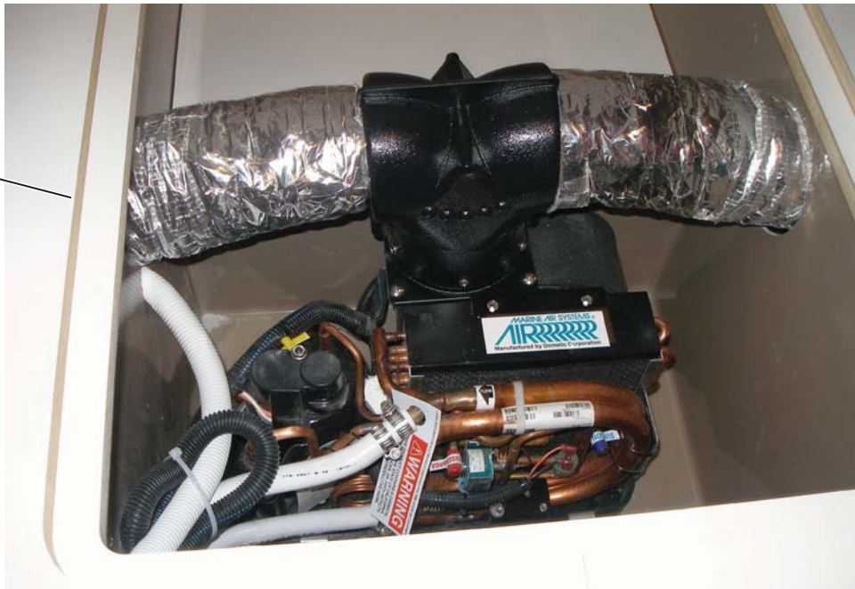
Air Conditioning Unit (8,000 BTU Unit)
