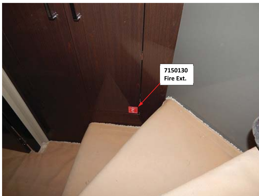
Figure 2-9 – Bottom of Port Side Storage at Entrance to Master Stateroom
