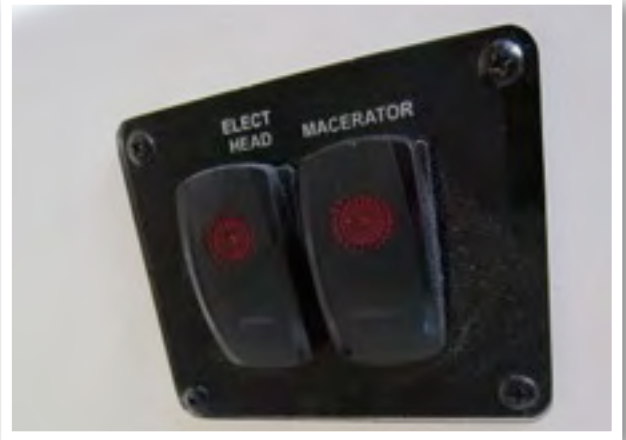
Toilet & Macerator Switch Located on Sink Cabinet
