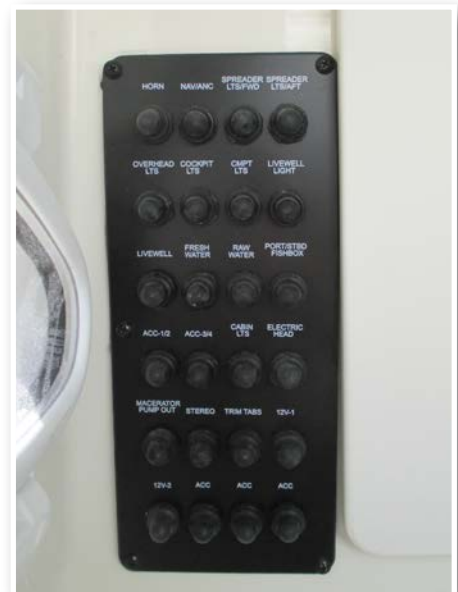
Main Breaker Panel
