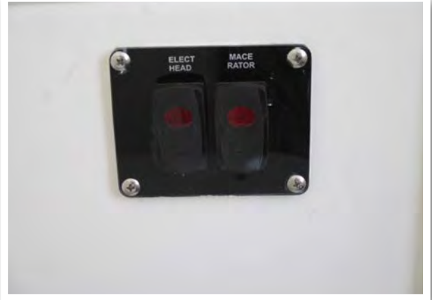
Toilet & Macerator Switch Located on the Starboard Aft Wall of the Console
