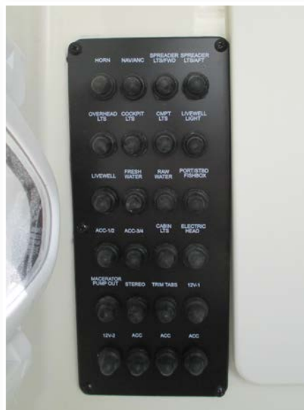
Main Breaker Panel
