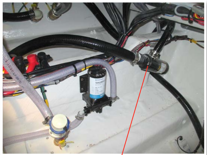
Starboard Macerator Pump
