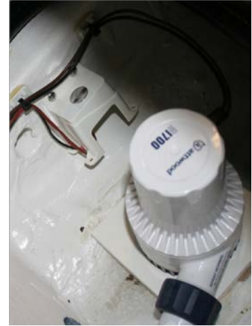
Aft Bilge Pump and Float Switch
