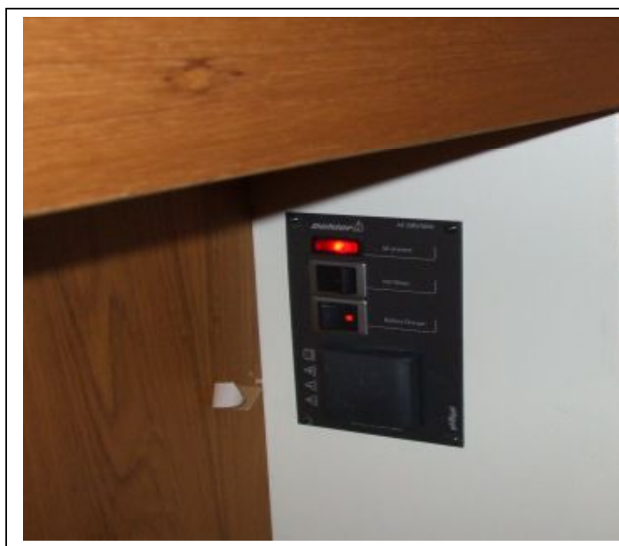
FIGURE 14: SHORE CONNECTION PANEL
