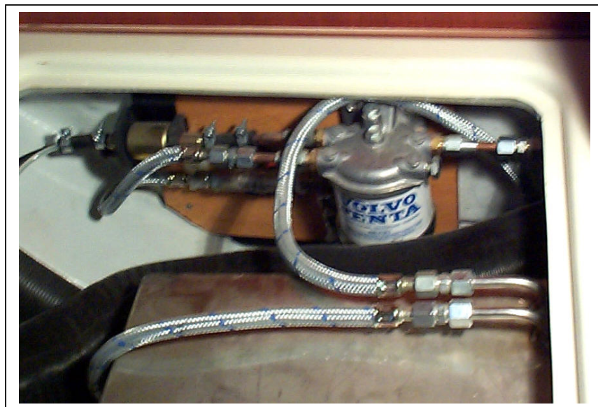
FIGURE.: DIESEL TANK
