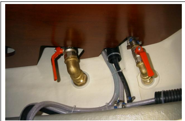
ABB.: RAPID SHUT OFF VALVE – WET AREA
