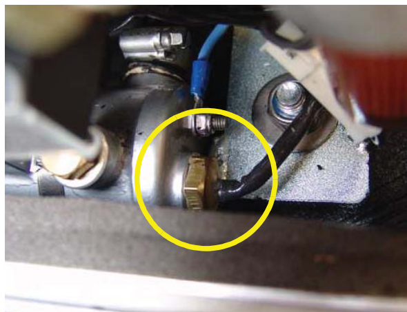
Fig. A.3.7-4: Thermo-sensor raw water in
