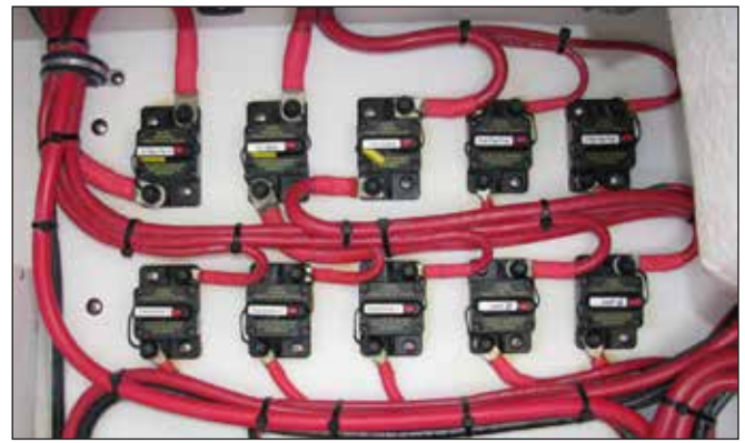
Heavy Duty Main Circuit Breakers
