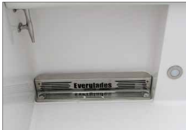
Typical Scupper Drains & Drain Rail
