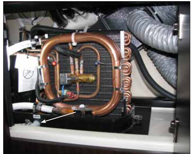
Typical Cabin Air Conditioning Unit & Condensation Pan Drain
