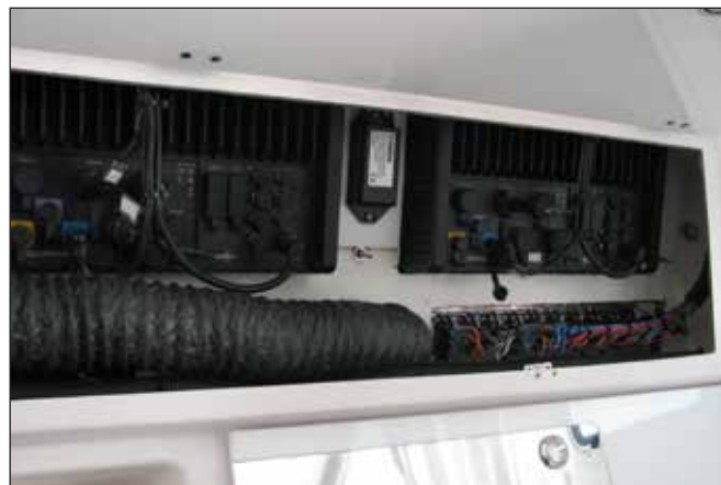
Upper Helm Access Compartment
