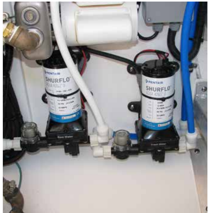
Fresh Water Pump & Strainer
