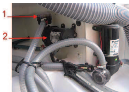
Location: Cockpit locker
