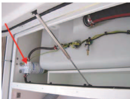
Location: petrol tank compartment
