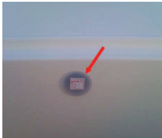
Extinguisher access hole - Compartment tank - Petrol
