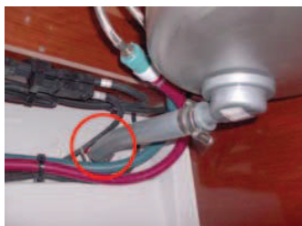
Drainage Galley sink
