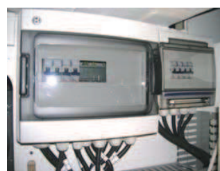
Circuit breakers (Ref 4) AC elements Air conditioning
