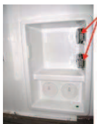
AC socket (Ref 1) House (Lower) & Air conditioning (Upper)
