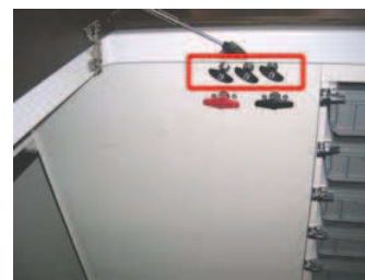
Remote shut-off pull handle - Diesel oil supply valve (Engine & Generator) (Ref 3)
