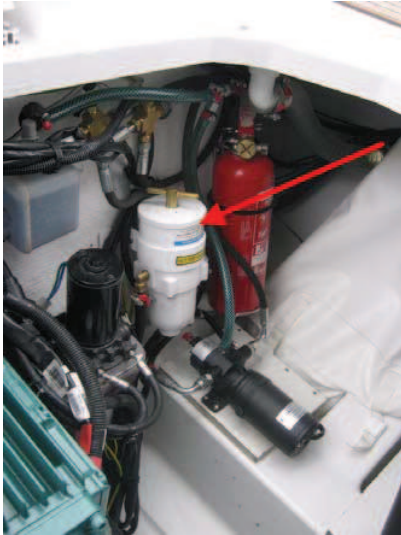
Diesel oil decanter valve
