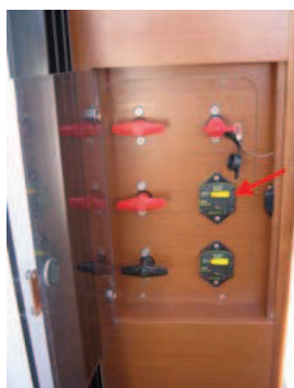
Windlass circuit breaker 90A
