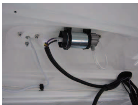
Location: Compartment - Roof
