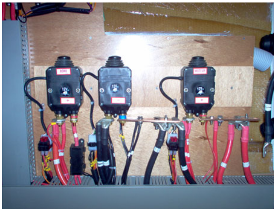
Access by trapdoor in aft cabin
