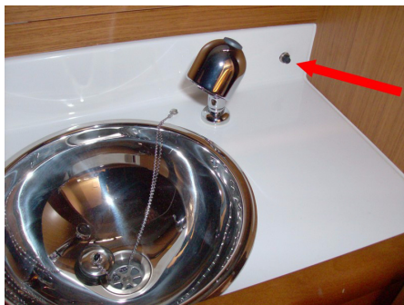
Control draining pump for shower
