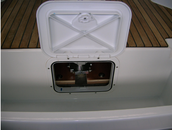
Inspection hatch - Cockpit aft
