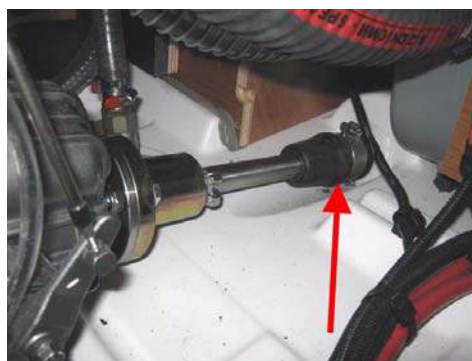
Access: Port aft cabin
