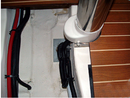
Mast harness exit at the stanchion base
