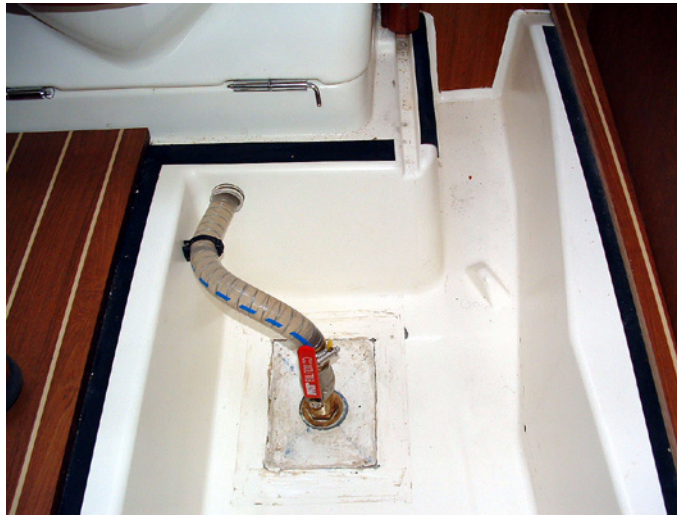
Thru-hull fitting with engine water inlet valve
