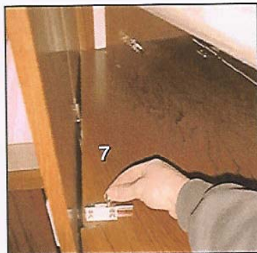
7- Unlock the bolt on the upper berth.
