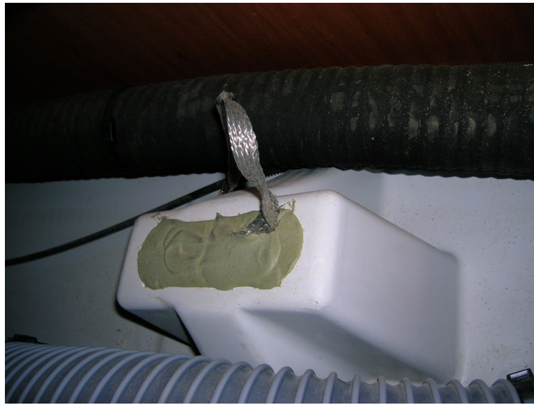
Access: Starboard aft cabin
