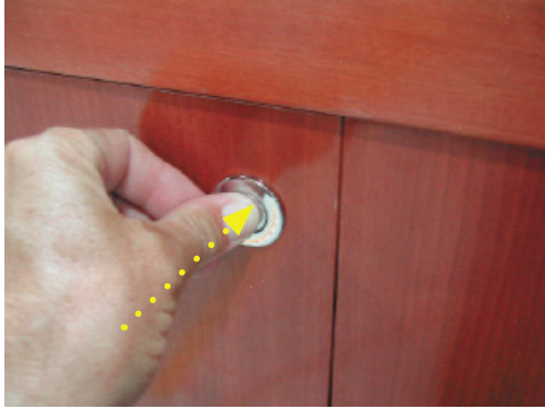
Releasing the door using the push-lock
