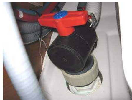
Thru-hull seacock
