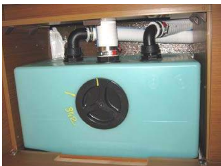
Holding tank Capacity: 80 litre Location: in each bathroom
