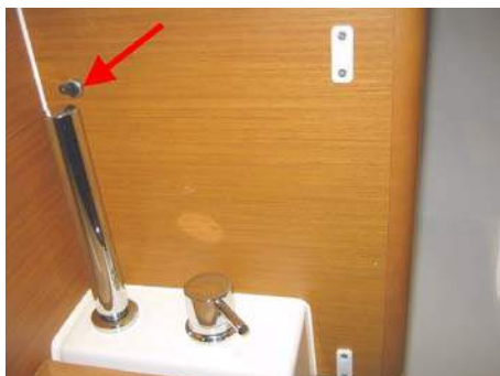
Drainage pump control
