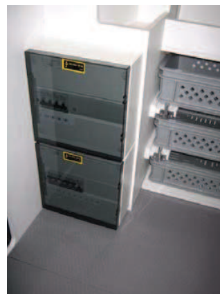
Circuit breakers - AC elements (Shore & Air conditioning) (Ref 3)
