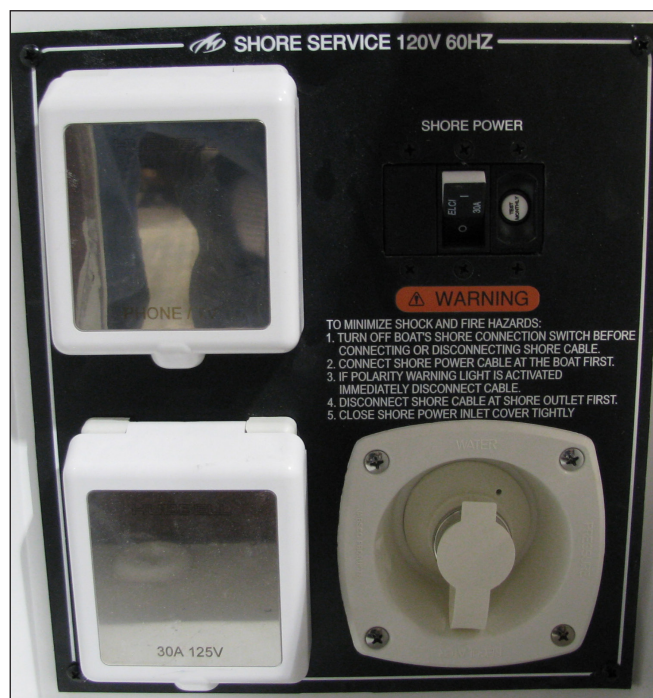
275/295SY 120 Volt Shore Inlet Panel With ELCI
