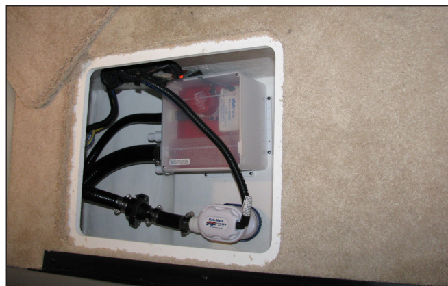
275/295SY Mid Berth Bilge Access Hatch
