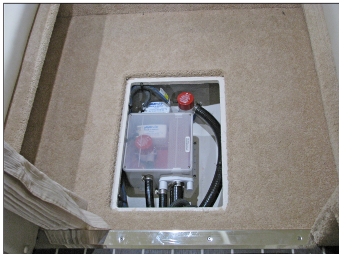
315SY Mid Berth Bilge Access Hatch
