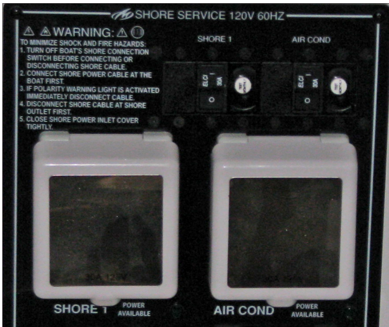
315SY Inlet Panel With Air Conditioning Option - ELCI Circuit Interrupter/Circuit Breakers
