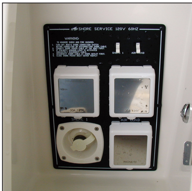
Shore Water Connection
