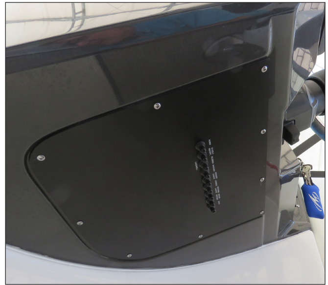
Helm Circuit Breaker Panel
