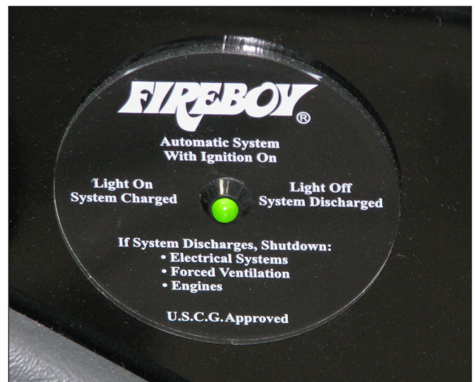
Typical Fire Extinguisher Panel In Helm
