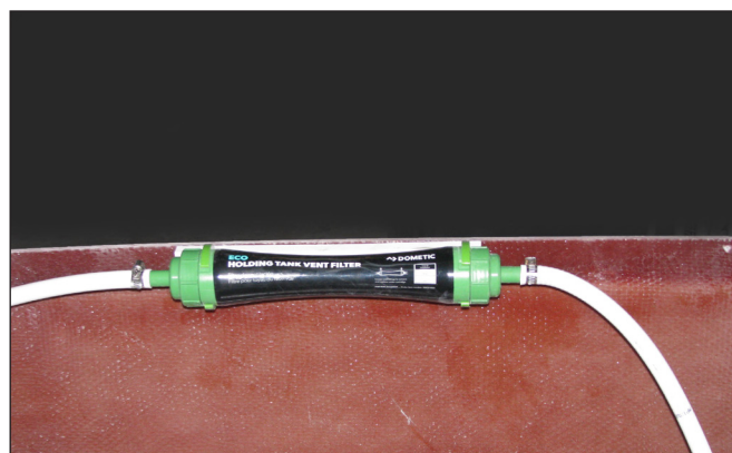
Typical Holding Tank Vent Filter
