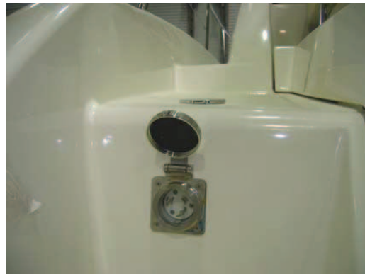
Shore power socket 32A - 220 V
