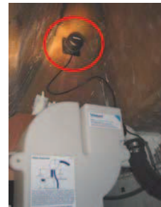
Gyrocompass Location: Cockpit locker
