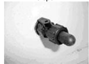
Lever on the aerator fitting is open
