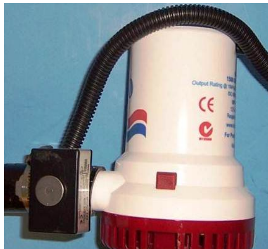
Bilge pump (typical)
