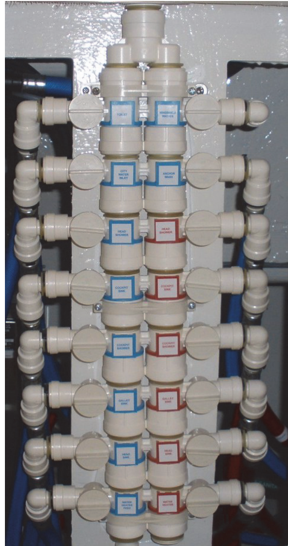
Water System Manifold (Typical)
