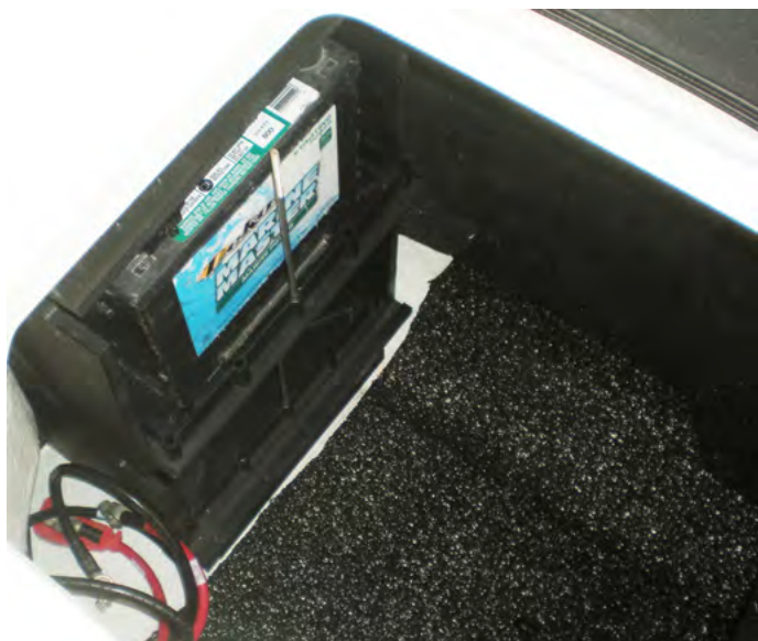
STACKED BATTERY SYSTEM
