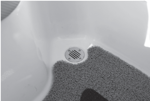
Figure B31: Liner Drain
