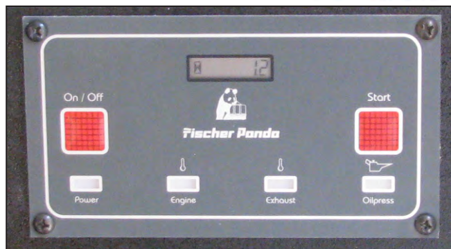
Typical Generator Control Panel
