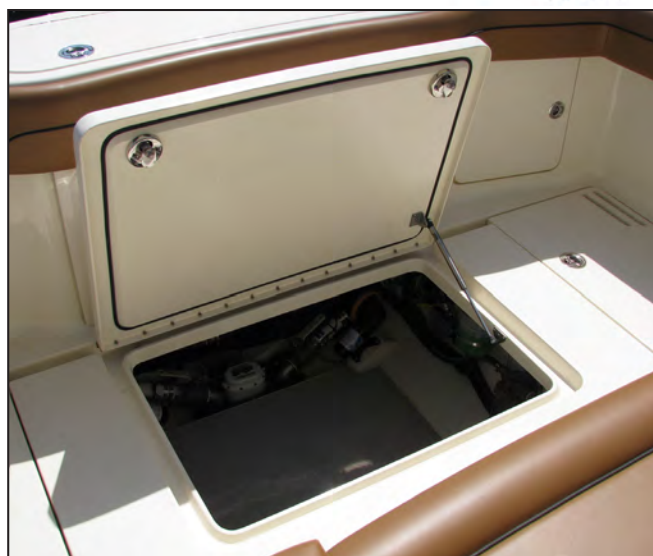
Aft Under Deck Systems Compartment
