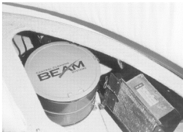
Wall Vacuum System (fig. 8.10.1)
