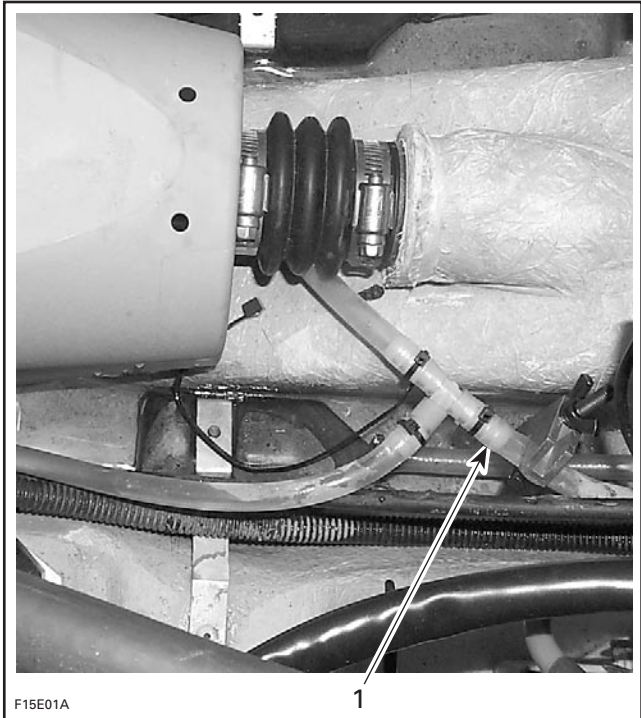
RFi MODELS — 787 ENGINES 1. Hose pincher installed on engine drain hose
