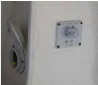
Breaker: Located starboard side of Hook Up.
