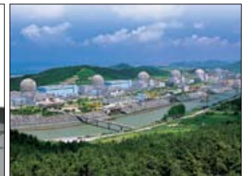
Emergency GenSets for Nuclear Power Plant
