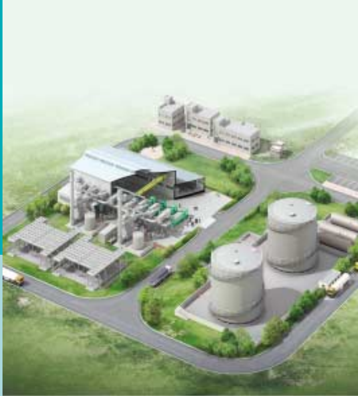
20 MW HiMSen Engine Diesel Power Plant (9H25/ 33 X 8 Sets)
